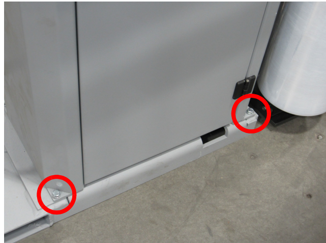
Figure 1 - 1 Tower to Base Bolts (2 of 4 shown)
