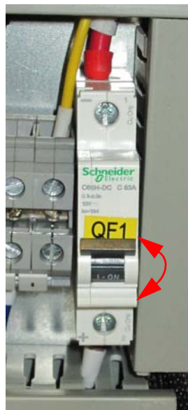
Figure 4 - 4 Main Disconnect
