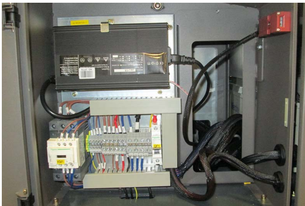
Figure 5 - 4 Right Side Electrical Enclosure
