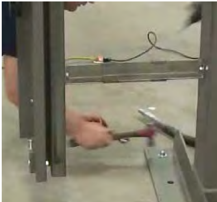
Figure 1 - 7 Installing Anchors
