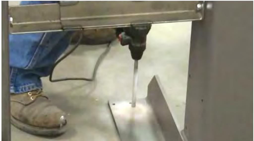
Figure 1 - 6 Drill Mounting Holes
