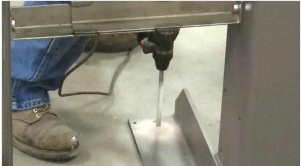
6. Pound in the 10 Red Head Anchors. The length of the anchors depends on the thickness of the concrete.
