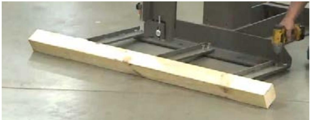
5. Using a hammer drill, drill the mounting holes in the floor with the correct drill bit to match the mounting hardware.
