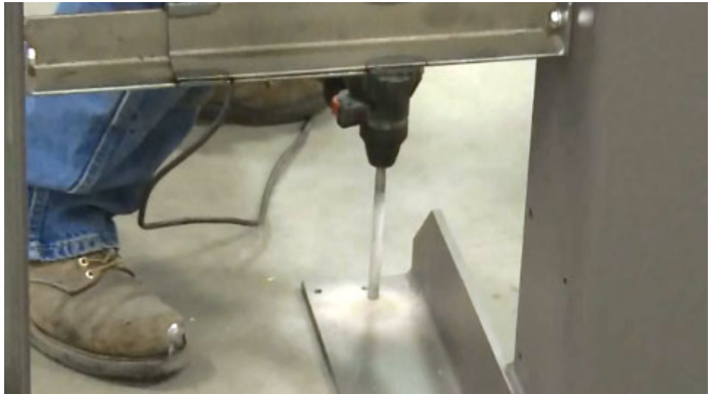
Figure 1 - 6 Drill Mounting Holes
