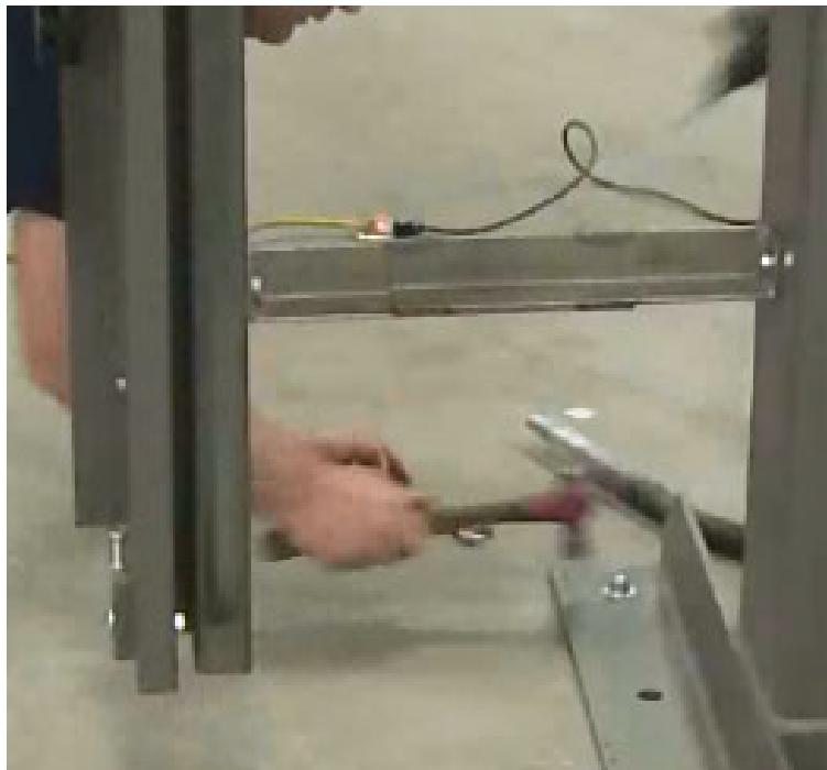
Figure 1 - 7 Installing Anchors
